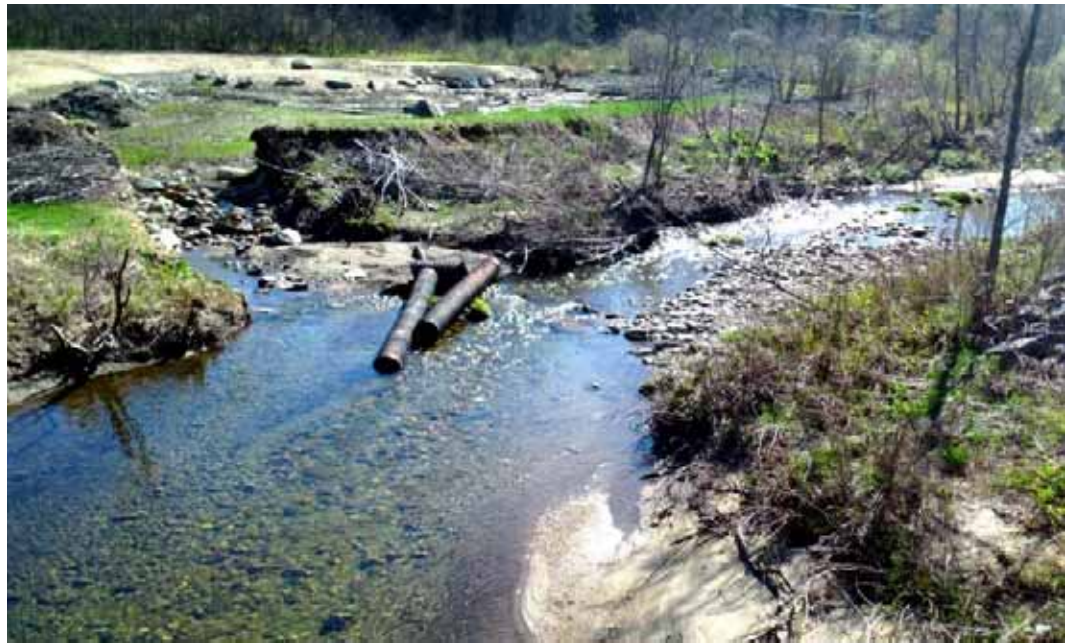
This Mt. Holly pond (top of photo) was constructed in the floodplain. During Irene the stream captured the pond releasing a surge of water and sediment downstream. Photo by Mike Winslow.
