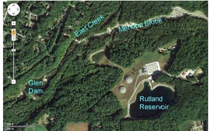
Emergency measures to protect the Rutland water supply led to later sediment build-up in Glen Dam, a hydropower source. Affected parties worked together to go back and correct the problems.
