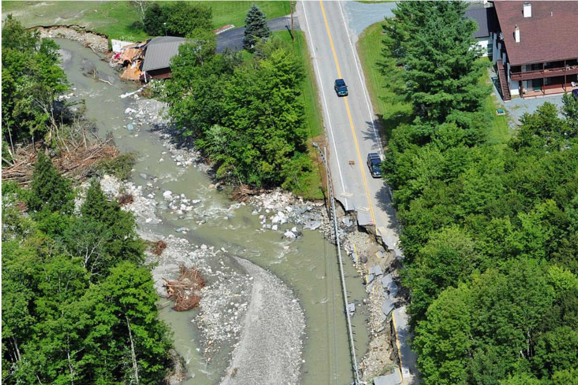
Irene left widespread destruction in its path, destroying roads and bridges like these along Route 100. Photo by Mansfield Helijflight.
