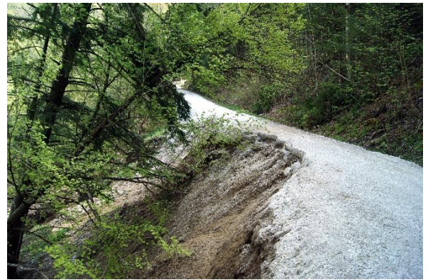
Upper Cold River Road in Shrewsbury washed away during Irene. Continued water seepage from the nearby hillside poses a significant construction challenge for this dirt road. Photo by Lori Fisher.
