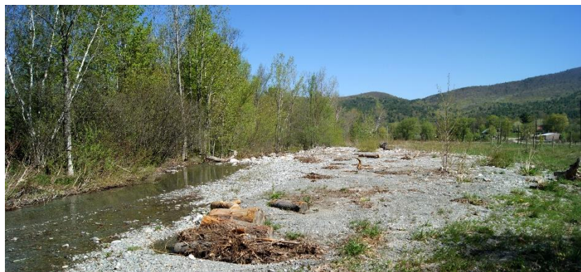
A berm along the right bank of Gully Brook (far left of photo) was removed prior to the storm providing the river additional flood storage capacity. Photo by Lori Fisher.
