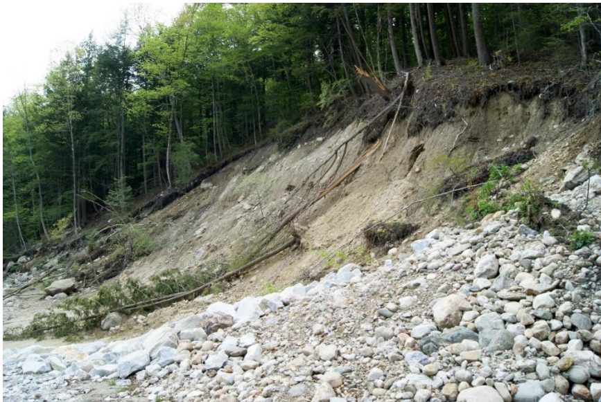
Landslide damage from Tropical Storm Irene along the Cold River. Photo by Lori Fisher.
