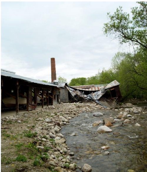
The former Vermont Tubbs furniture factory in Forestdale. The factory was destroyed when the Neshobe River escaped a berm on the left bank. Photo by Lori Fisher.
