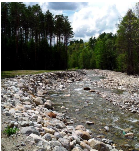
The Mendon Brook near the Rutland water intake jumped the left bank near this spot threatening the intake. Photo by Lori Fisher.
