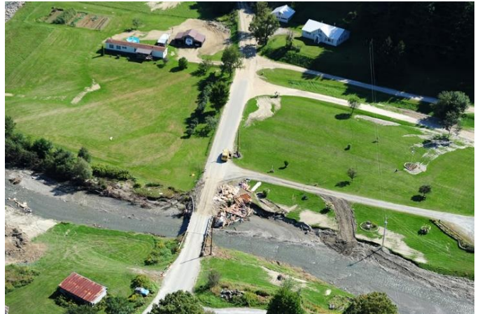
In Bridgewater Corners a house washed up against the bridge, blocking water and threatening to wipe out the bridge. Photo by Mansfield Heliflight.
