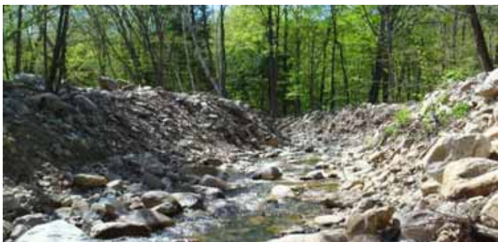
Berms along Homer Stone Brook gave local residents a sense they were safe from the water, but the brook escaped the berms during Irene. Photo by Mike Winslow.
