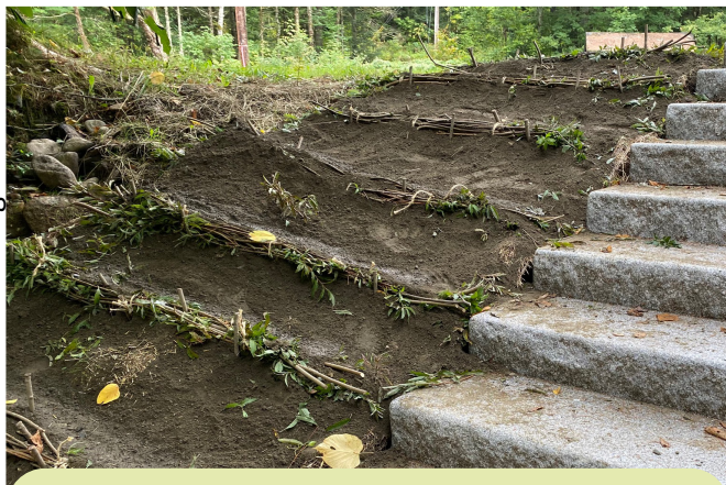
Section of a fascine > staked into a steep bank.
