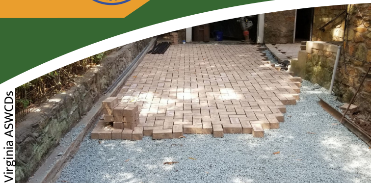
Laying interlocking permeable paver blocks.
