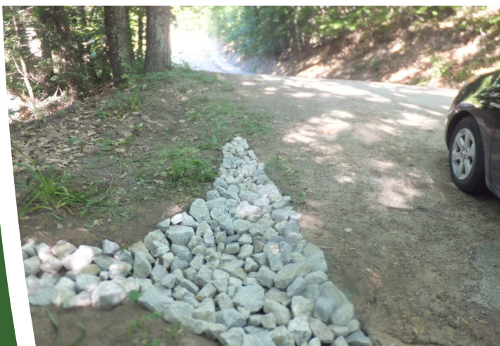
Turnout stabilized with angular rock .
