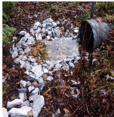
Small rock apron at culvert outlet.
