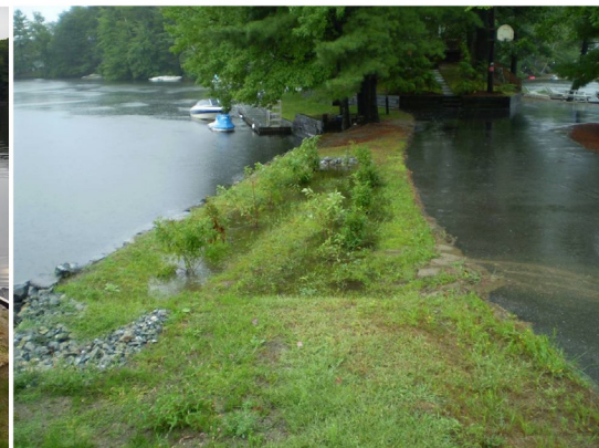
After: Meandering vegetated swale installed with erosion control slows and treats road runoff, allowing sediments to settle and pollutants to be filtered.
