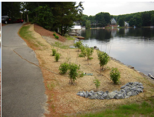
After: Meandering vegetated swale installed with erosion control slows and treats road runoff, allowing sediments to settle and pollutants to be filtered.
