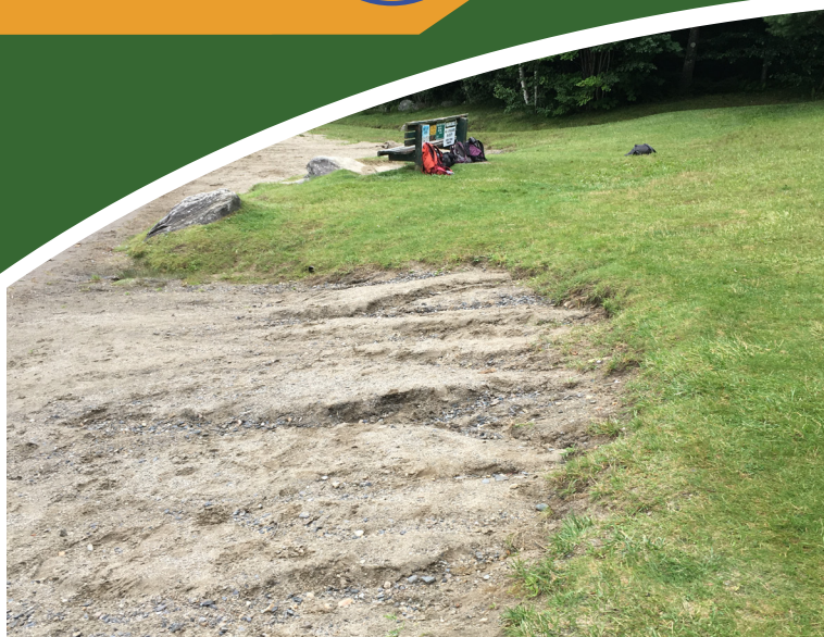
BEFORE: Lake Reponda beach in Wilmington, VT was undefined and eroding from upland stormwater runoff.
