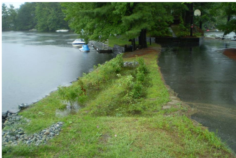
A vegetated swale at Lake Shirley, MA and open-top culverts at Lake Eden, VT access intercept road runoff.
