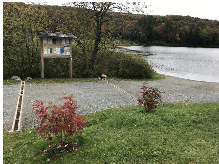
A vegetated swale at Lake Shirley, MA and open-top culverts at Lake Eden, VT access intercept road runoff.
