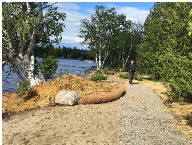
ADA compliant permeable geogrid and peastone pathway.
