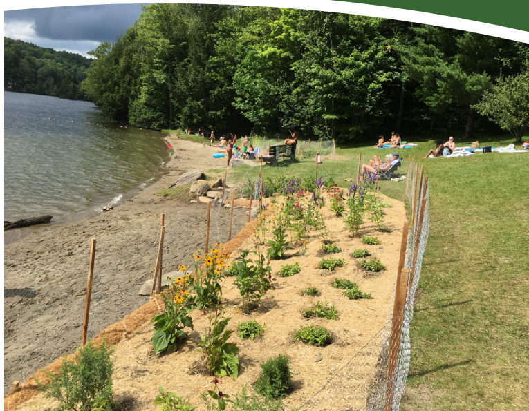
INSTALLATION: Stabilized with fiber coir rolls, erosion control blankets, native plantings, and stone step access.
