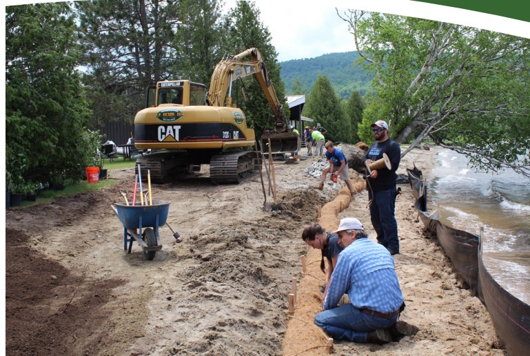
INSTALLATION: Erosion control with fiber coir rolls.
